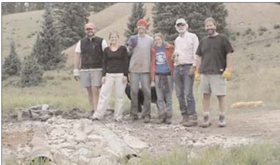
Eric Schlenker-Goodrich, Western Environmental Law Center; Rachel Conn, volunteers Ethan Timm, Lauren Kawa, Bob MacPhearson, and Allan Pasteris beside the French drain created to protect the Red River from erosion from ORVs
